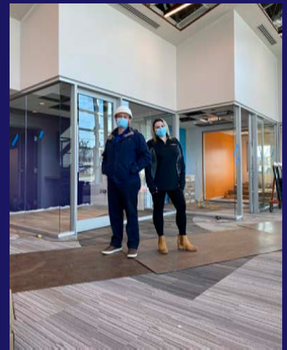
Dan DeAngelis, VP Facilities & Mikala Geurtsen, AVP Corporate Clerk & Project Manager, check in on progress at the new Washington St. Branch.
